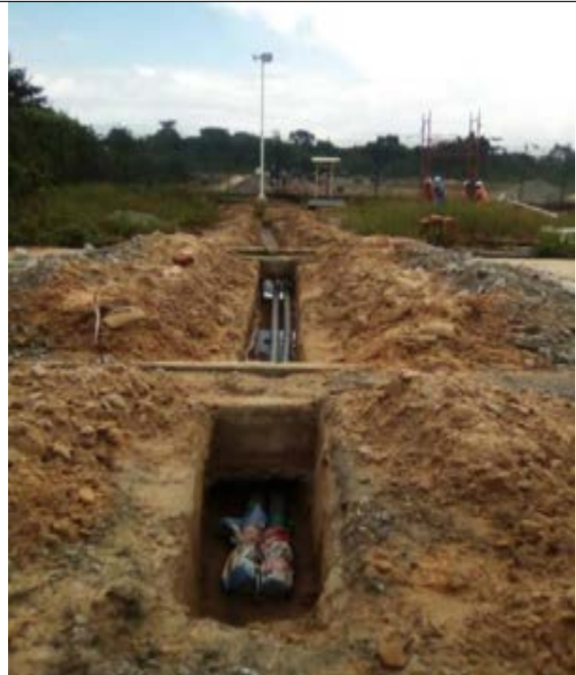
Fig 4.10: Pipes for cable road crossing
