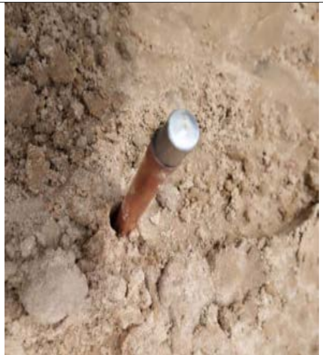
Fig 5.4: Earth rod in ground
