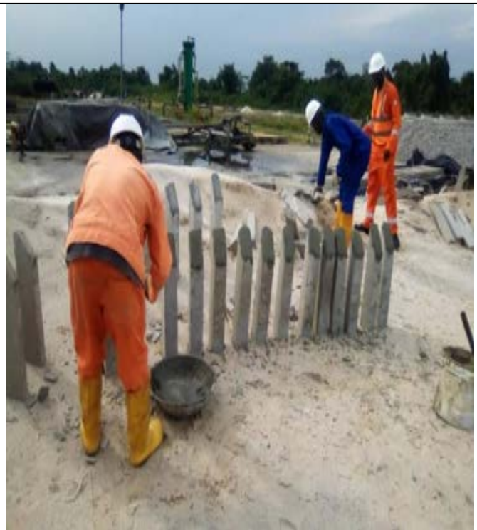
Fig 4.12: Casting of cable marker
