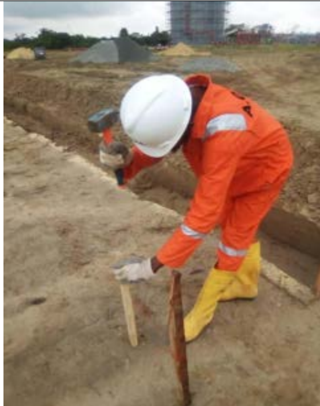
Fig 4.1: Perimeter lighting setting out
