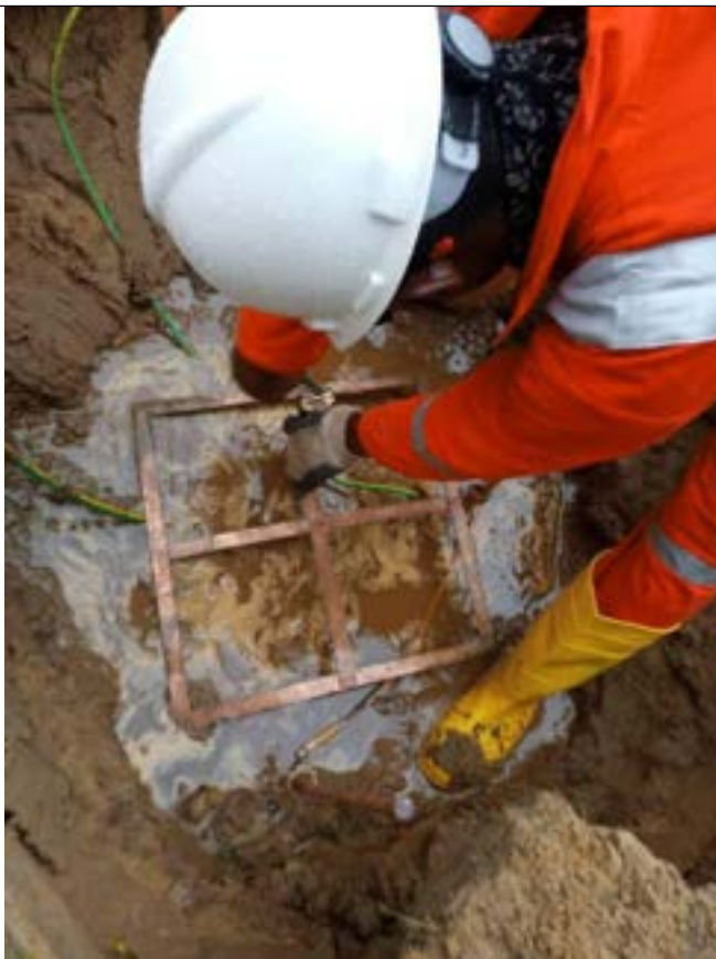
Fig 4.5: Copper earth mat installation
