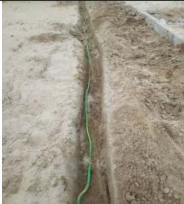
Fig 5.1: Excavation and cable laying
