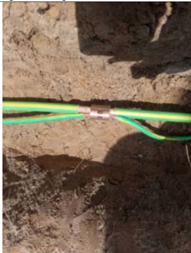
Fig 5.11: Bonding of earth grid with c-clamp
