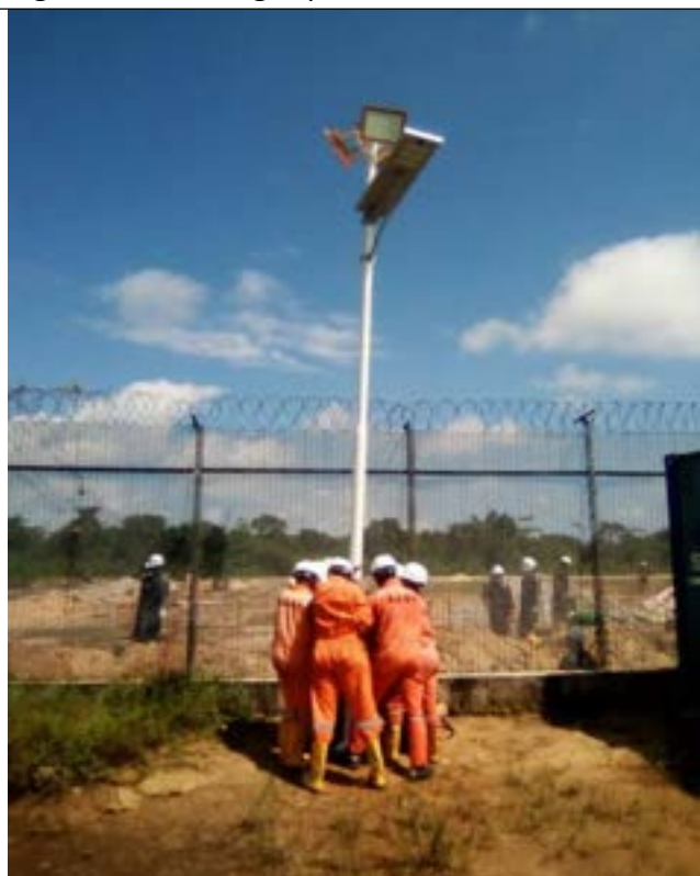
Fig 4.7: Erection of light pole with solar and main light fittings
