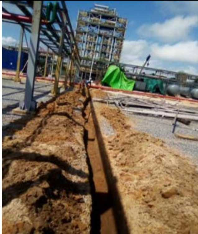
Fig 4.9: Excavation of cable route
