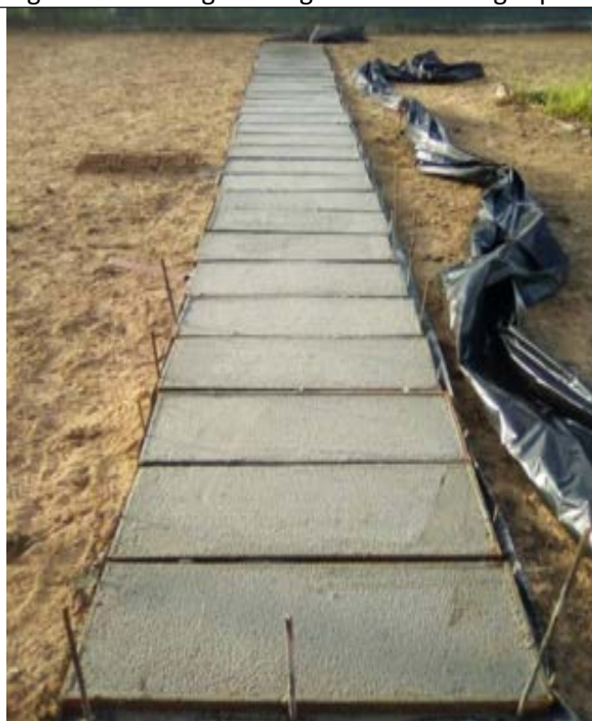
Fig 4.8: Casting of Cable slab
