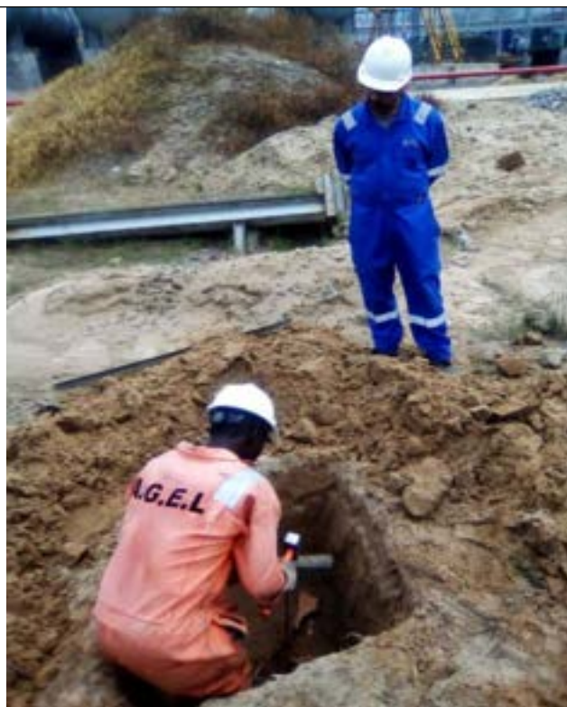
Fig 5.7: Earth rod installation process
