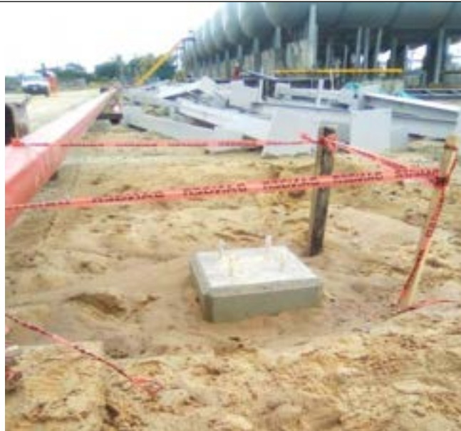
Fig 4.3: Prepared pole pedestal
