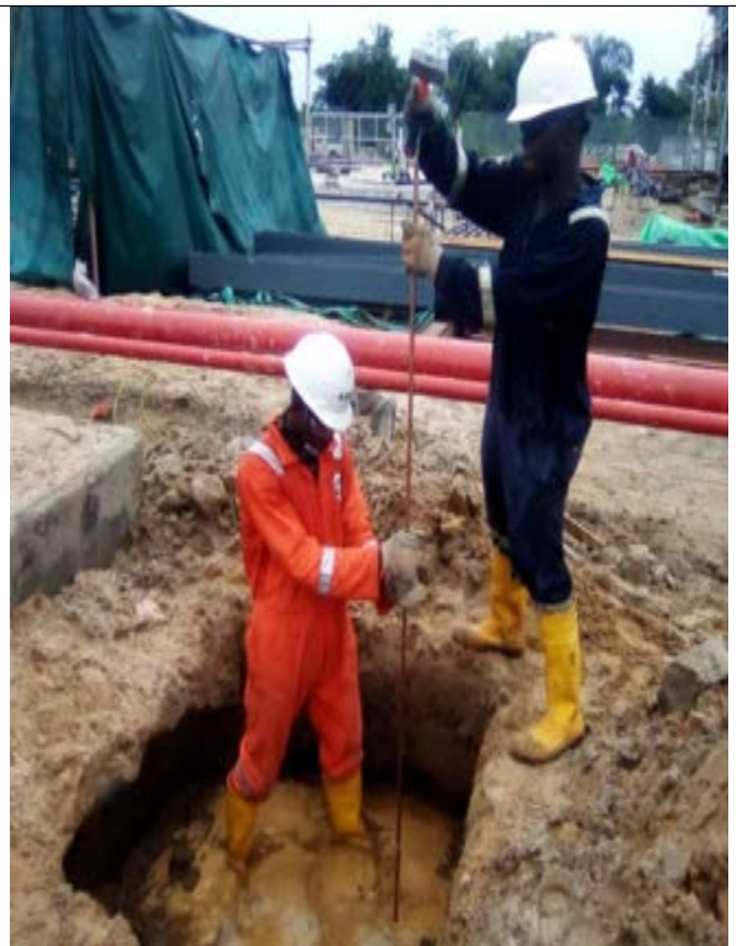
Fig 4.6: Earth rod installation
