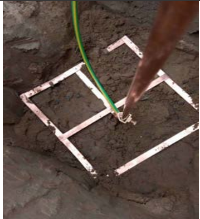
Fig 5.2: Earth mat installed
