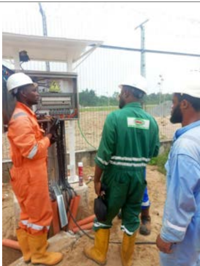
Fig 4.17: Testing of lighting panel
