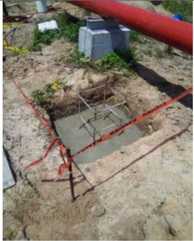
Fig 4.2: Casting of light pole base
