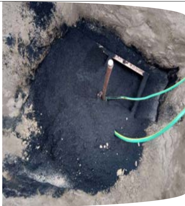
Fig 5.3: Copper cables connected to earth rod
