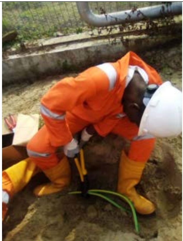
Fig 5.12: Cable bonding ongoing
