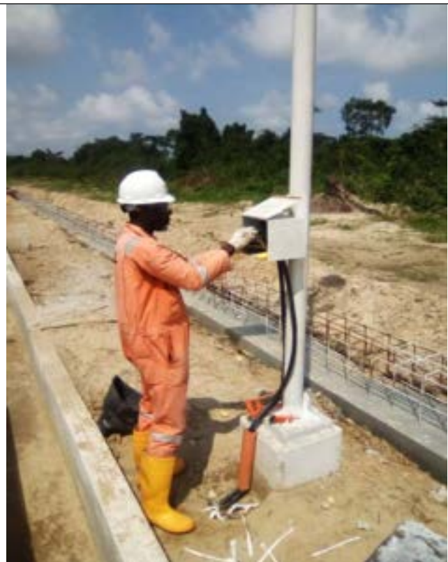
Fig 4.14: Termination of cabled in lighting JB
