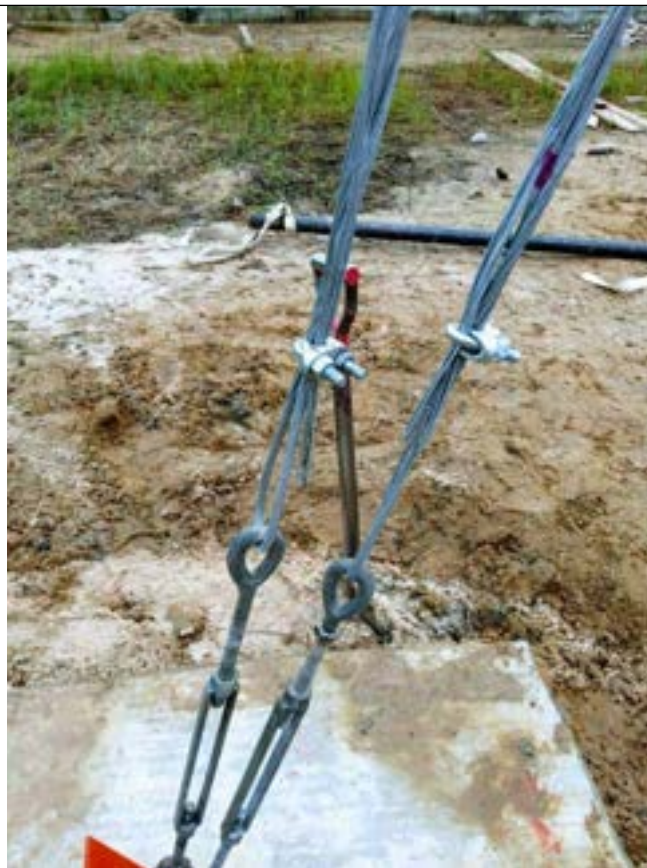
Fig 4.11: Mast guyed wires
