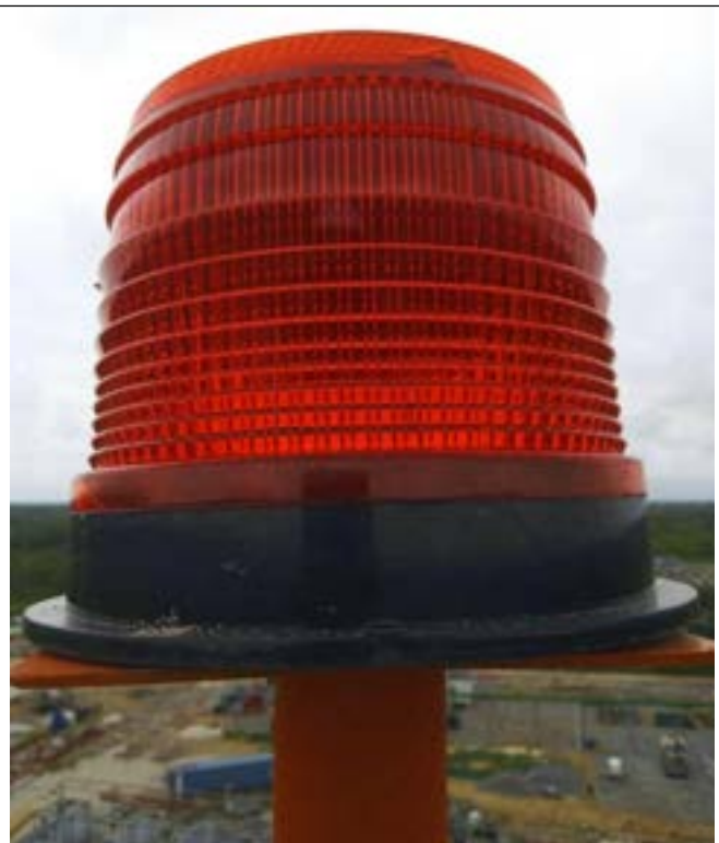
Fig 4.10: Aviation light on top of mast
