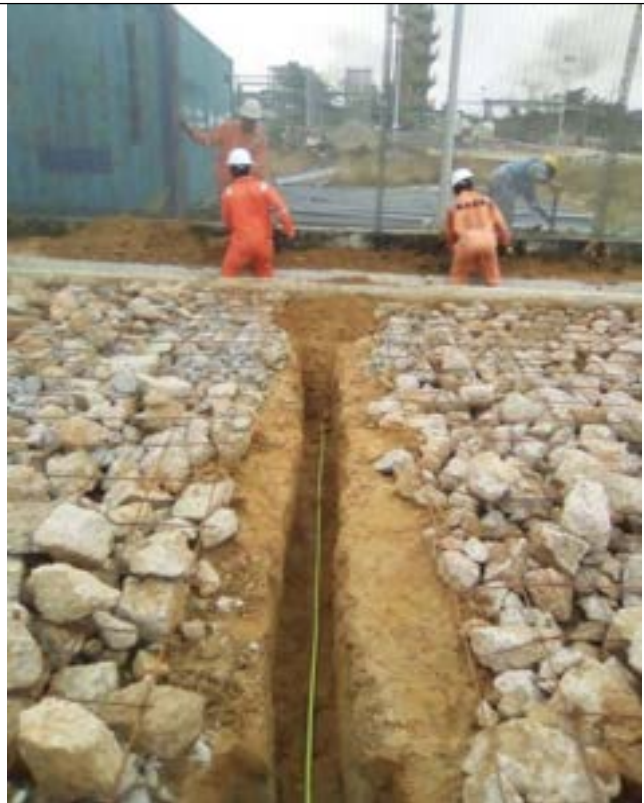
Fig 5.10: Cable laying on road crossing
