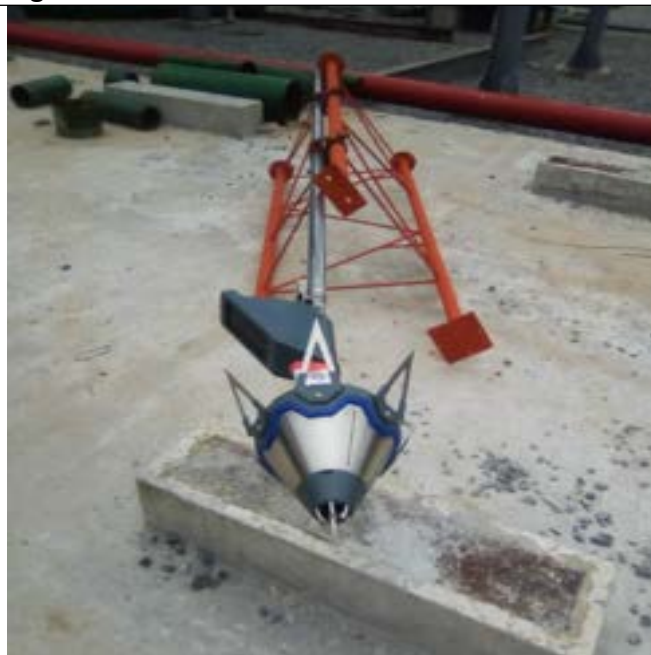
Fig 4.3: PREVETRON3® S60 ESE connected to mast member
