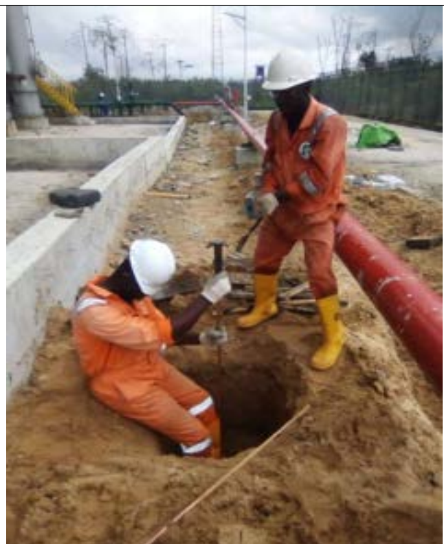
Fig 5.8: Driving down earth rod
