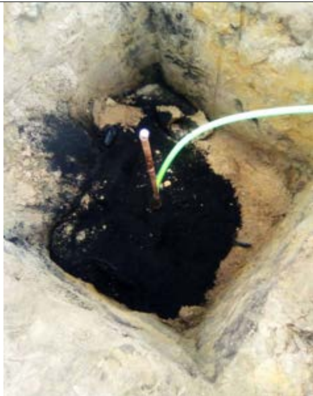
Fig 5.9: Earthing enhancement chemical
