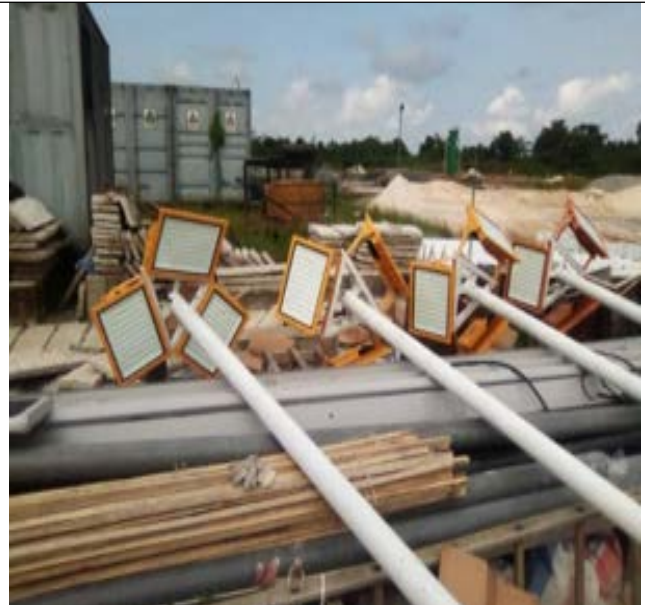
Fig 4.4: Light fittings prepared and terminated
