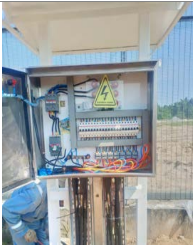
Fig 4.18: Connected lighting panel
