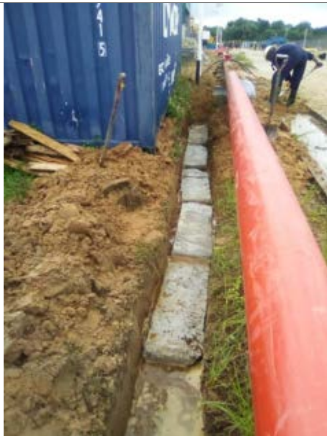
Fig 4.13: Laying of cable slab on cable way
