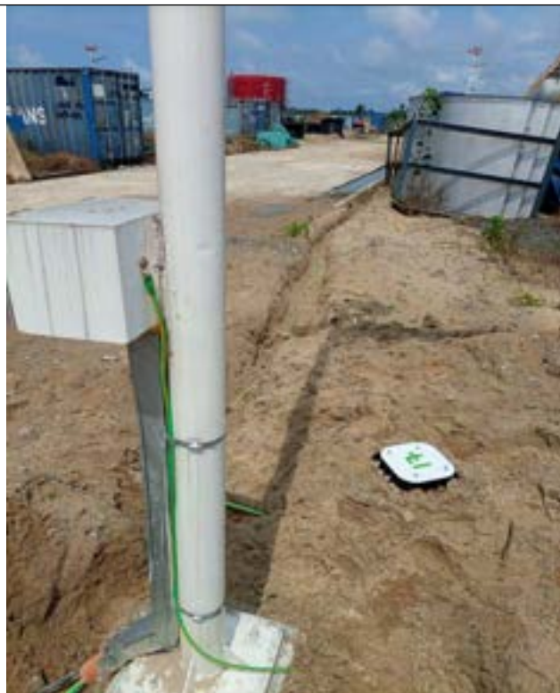
Fig 5.5: Termination of lighting pole to earth
