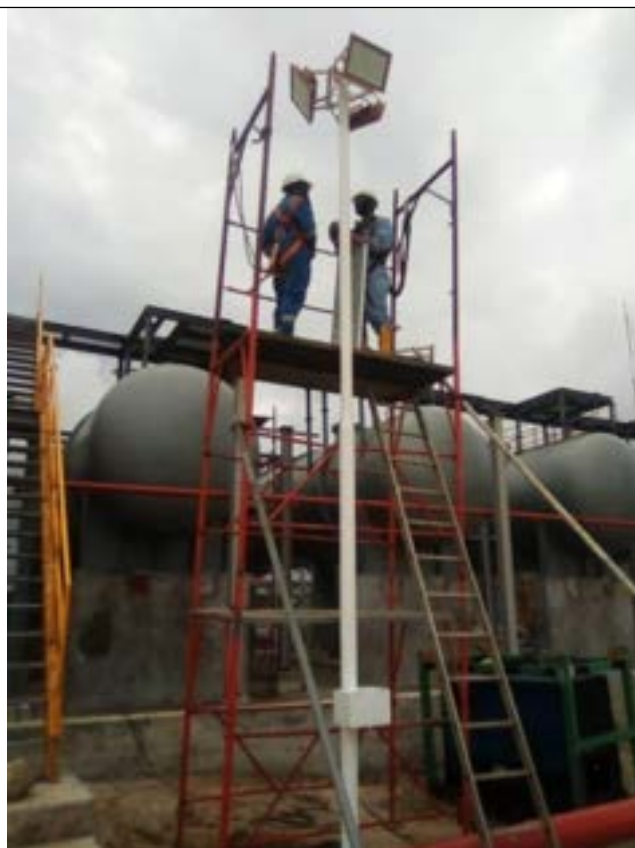
Fig 4.6: Mounting solar light on erected light pole
