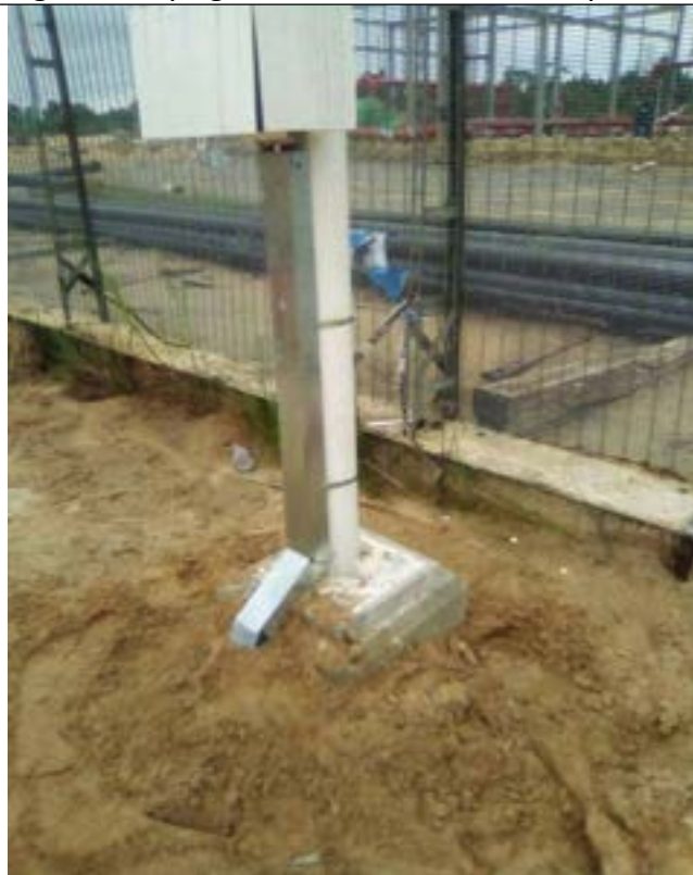
Fig 4.15: Light cables in cable tray and extra protection for JB
