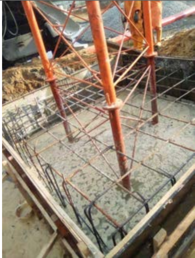
Fig 4.1: Mast foundation
