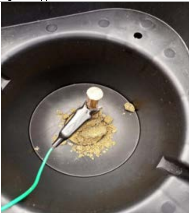
Fig 4.7: Earth rod outlet in chamber
